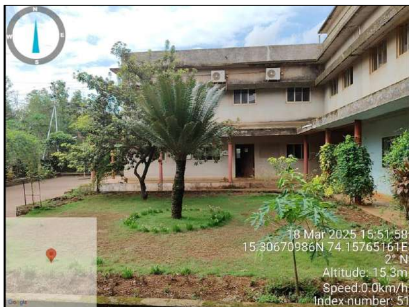
Greening in the Plant area
