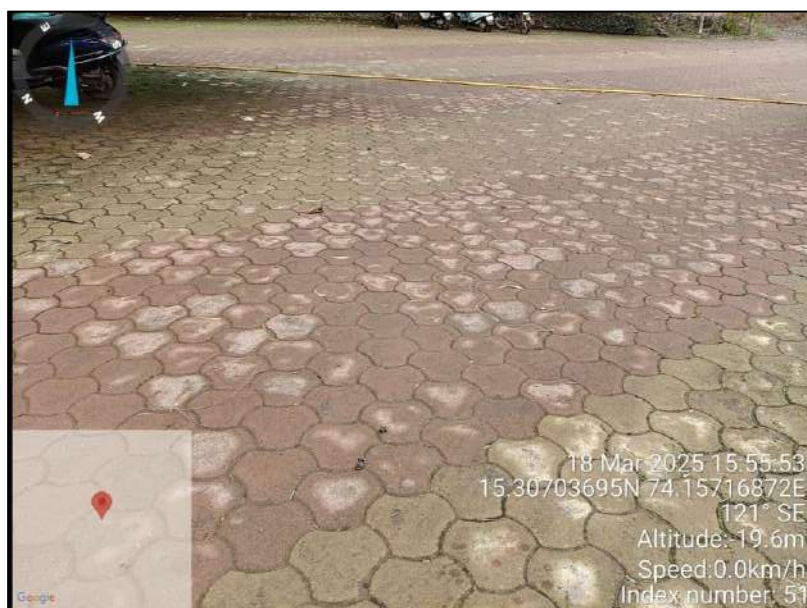
Paving within the Plant area
